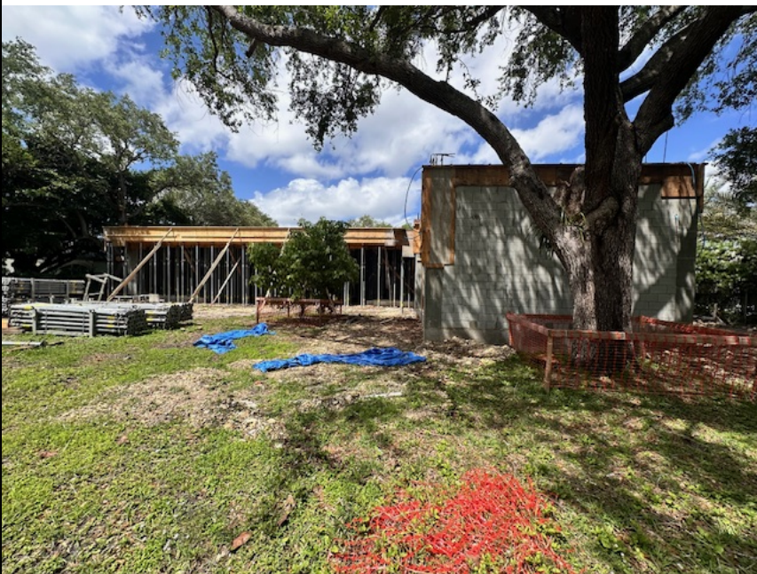
Photo Two Caption: REAR VIEW (04/14/2026)
