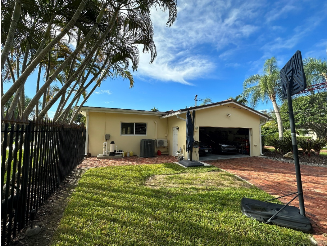
View of two-car garage with HVAC unit
