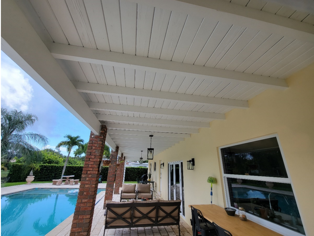
Exterior view of home with wood ceiling
